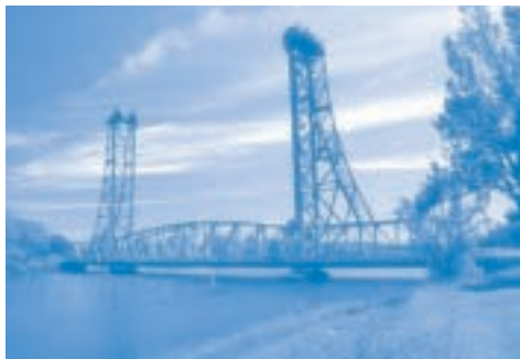
Light bridge on old canal, Welland Canal
