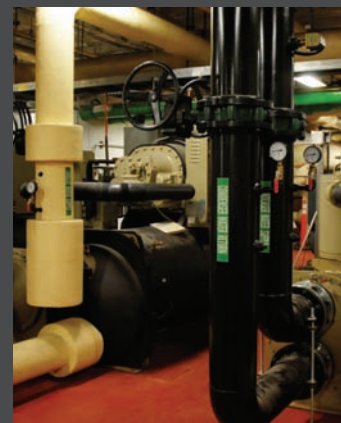
Great-West Life uses Five 400 Ton Trane R134a High Pressure Chillers
