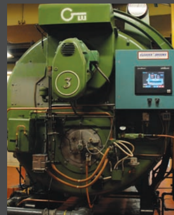
One of three 300 Hp Cleaver Brooks Boilers at Great-West Life
