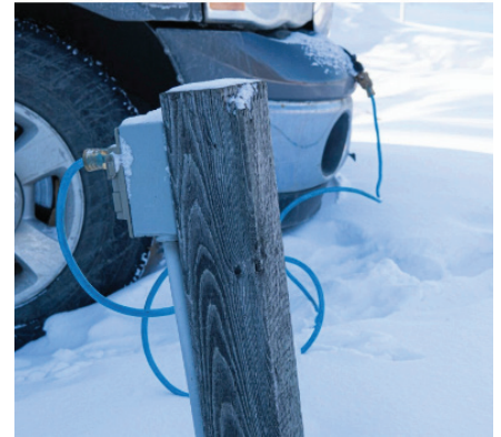
Figure 14B: Perform annual inspection and testing of plugs and conduit, especially before winter.
