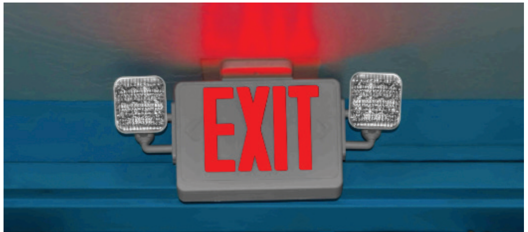
Figure 7D: Check exit signs, replacing failed lamps or batteries.
