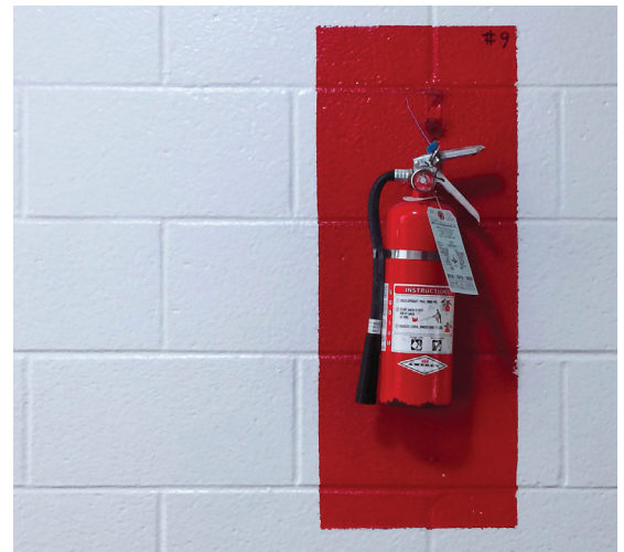
Figure 9A: Fire extinguishers should be inspected monthly and serviced annually.
