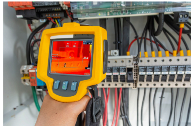
Figure 7A: Document thermal images and compare results over time.
