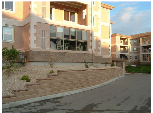
Figure 13A: Keep planting beds and lawns in good condition to stop soil erosion or displacement toward buildings.
